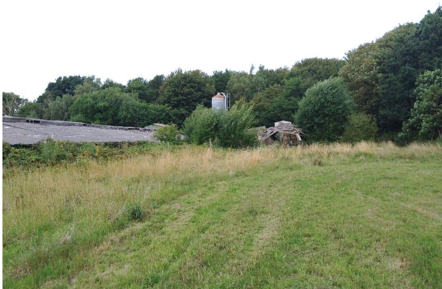
Photo 4 – Views towards the west and southeastern elevation of the shorter (derelict) existing agricultural building
